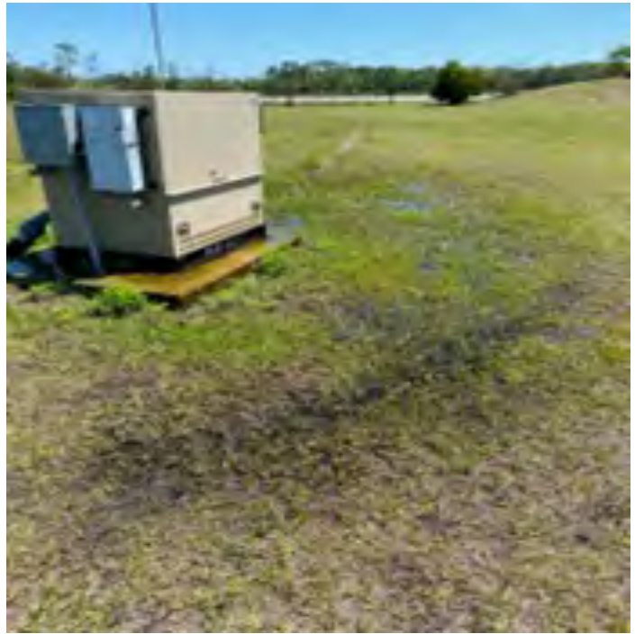
Irrigation Pump Repair
