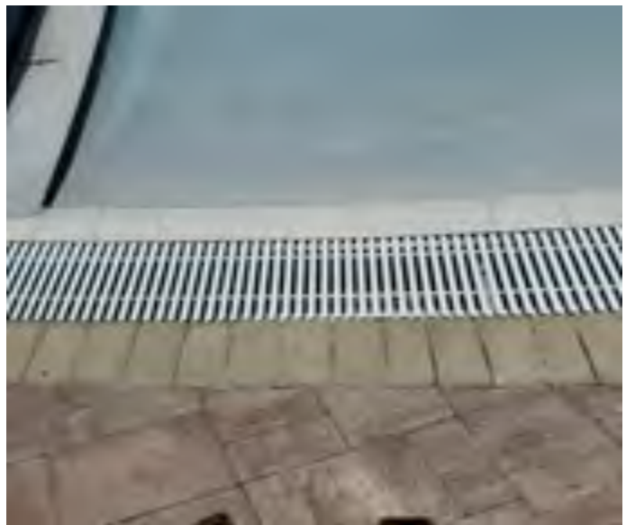
Entry Pool Tile Replaced
