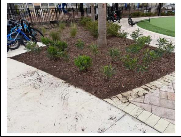
New Bushes Installed
