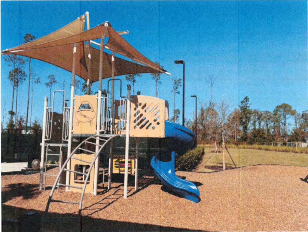
Playground in good condition, with no deficiencies.
