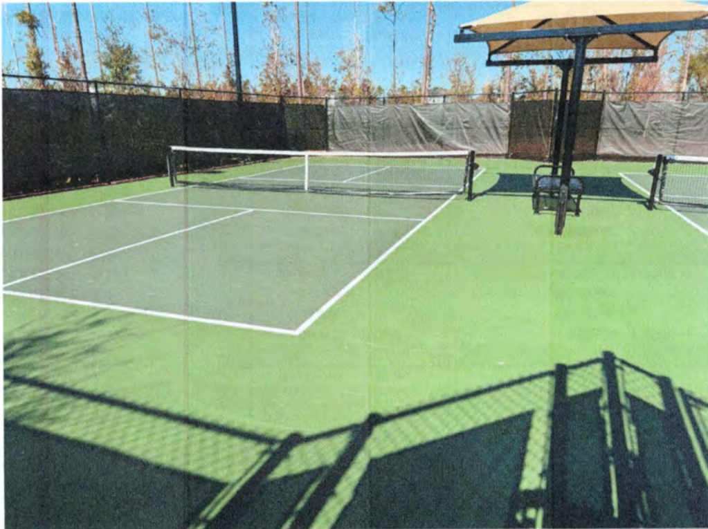
Pickleball Court in good condition, with no deficiencies.
