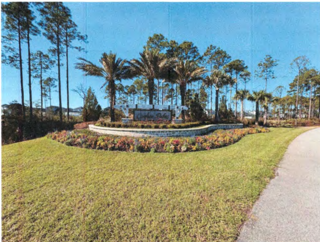
Entry monument no deficiencies.
