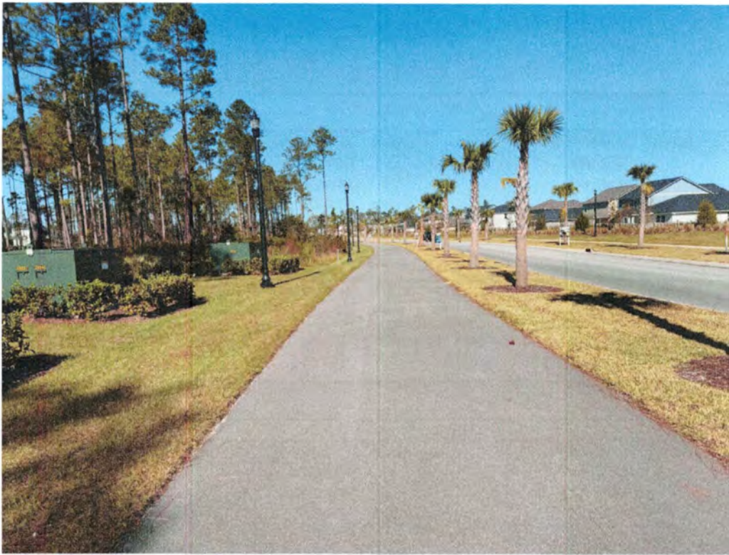
Multiuse Path in good condition, no deficiencies.
