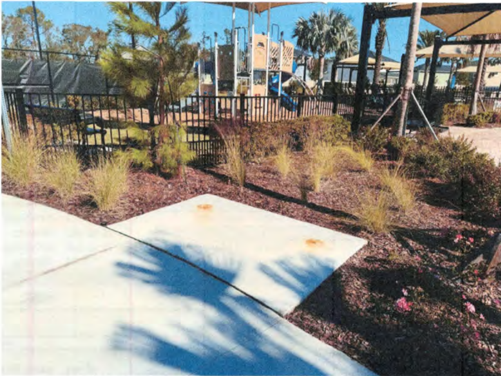
Missing bicycle rack at children's playground / putting green.
