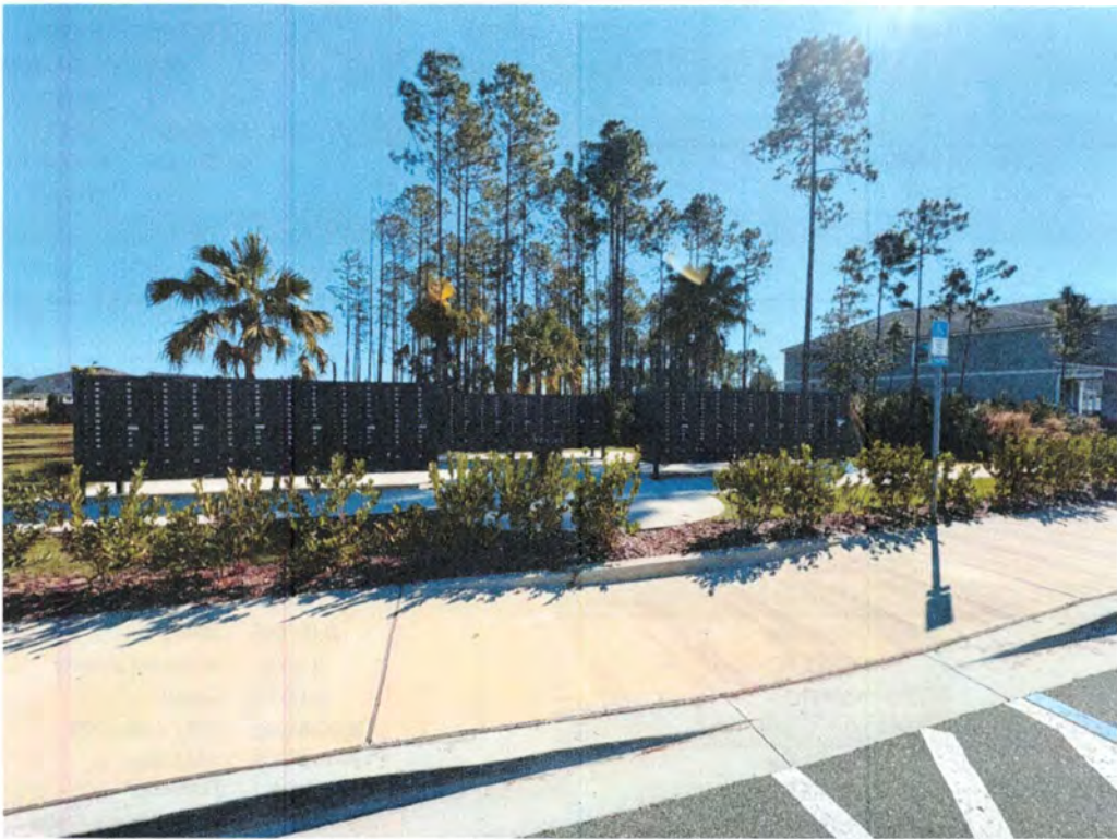
Mail kiosk at Cordova Palms and Bermudez Way in good condition, no deficiencies.
