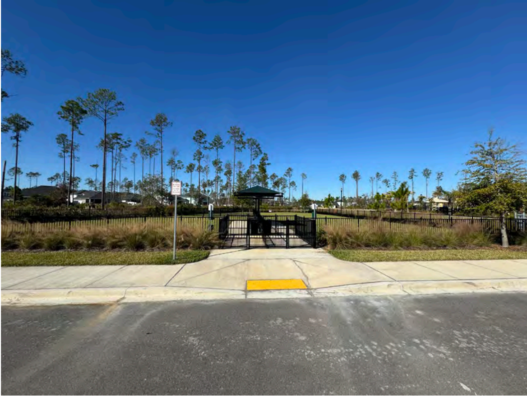
Dog park is in good condition, with no deficiencies.
