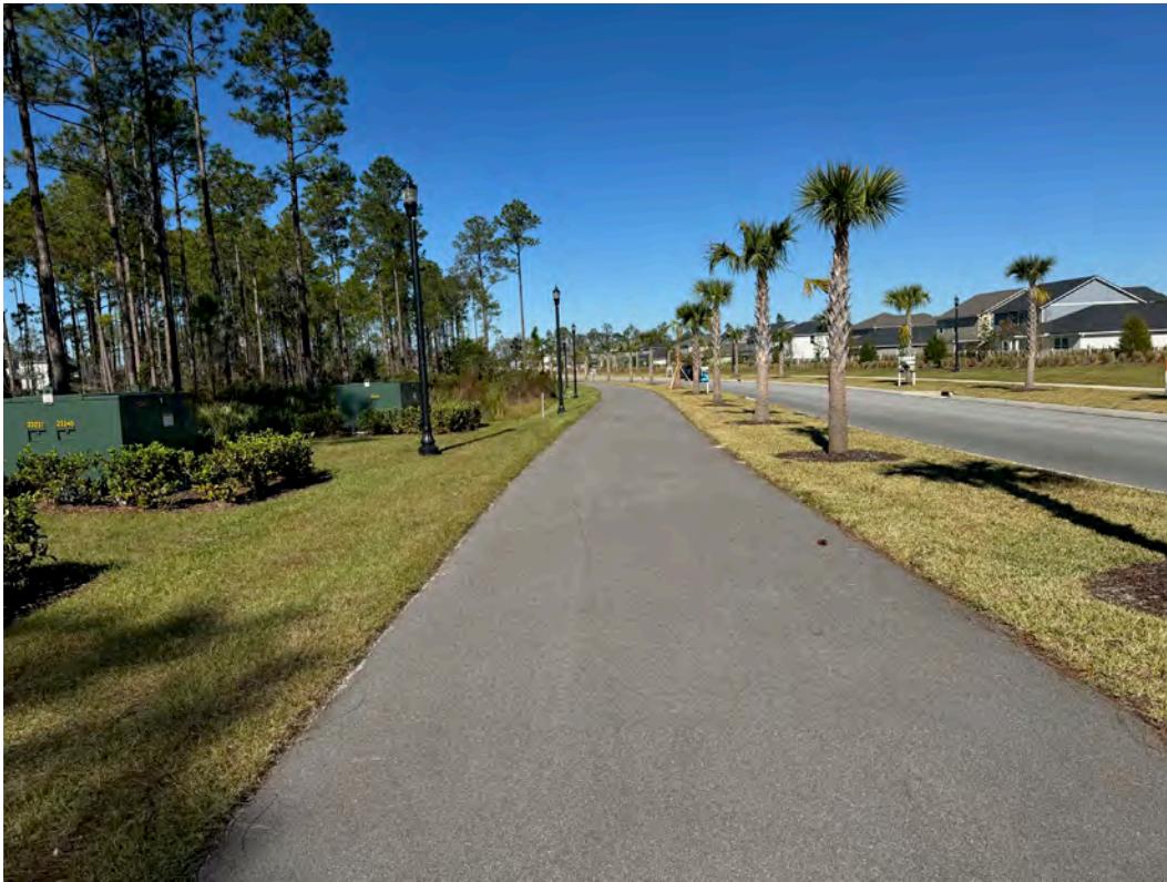
Multiuse Path in good condition, no deficiencies.
